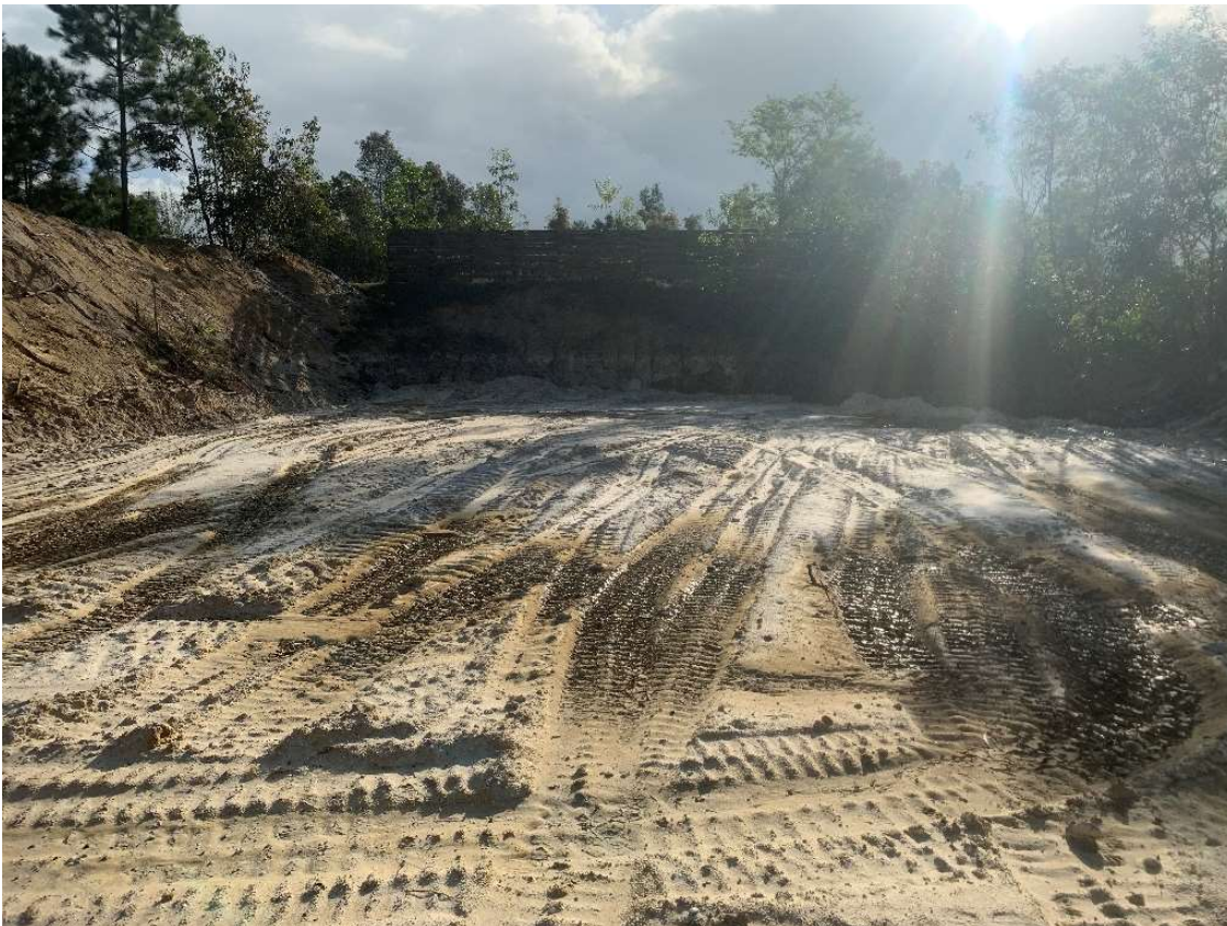
Reopened Bay 1B, looking east:
