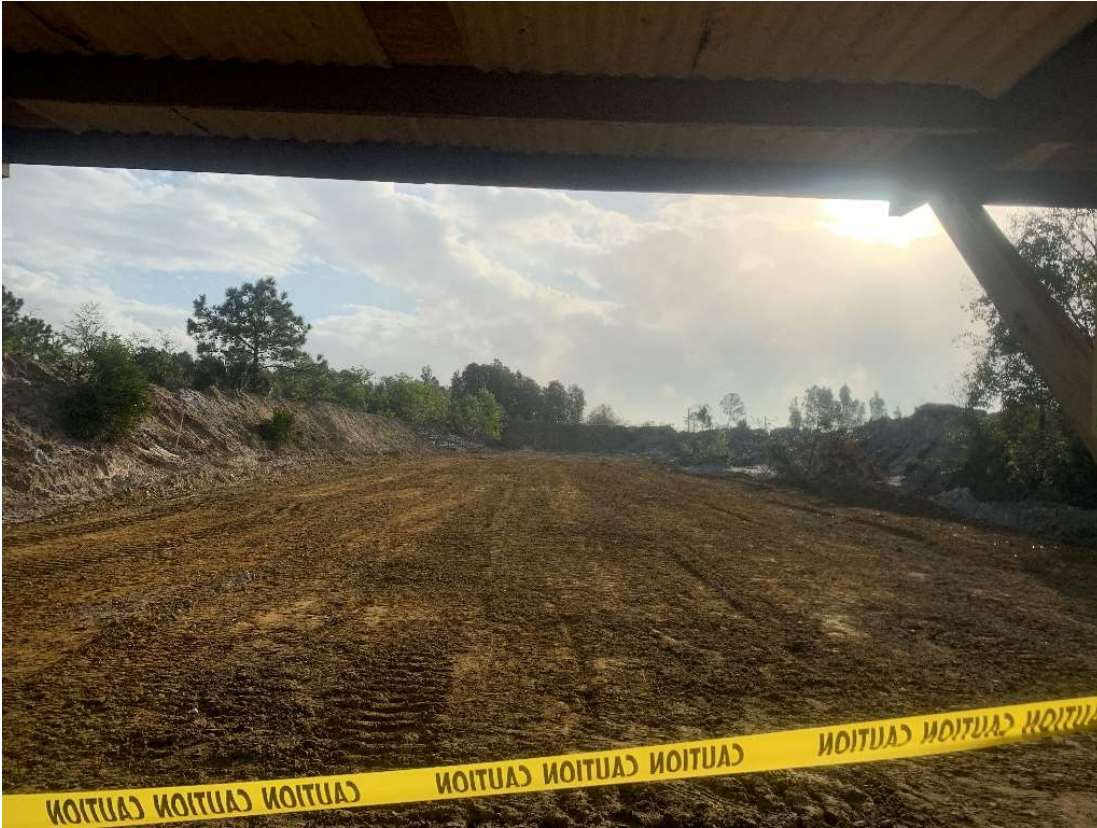
Reopened Bay 2, looking east:
